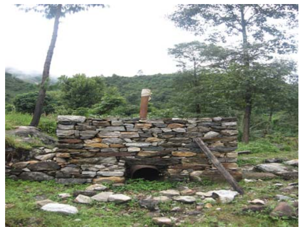
Advanced Alainchi Stack under construction
