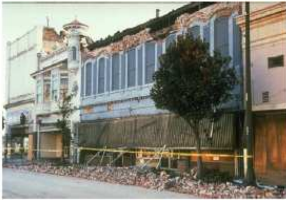
Watsonville, Loma Prieta Earthquake, 1989
