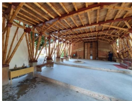
Figure 4: Bamboo structure for the school building
