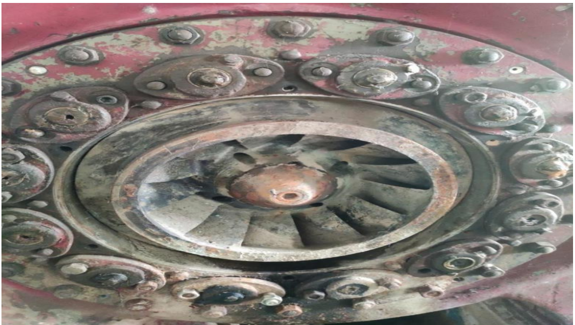
Photo 7: Existing Condition of the Turbine Runner
