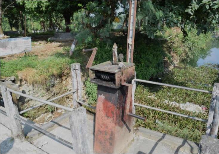
Photo 1: Main Intake Gate
