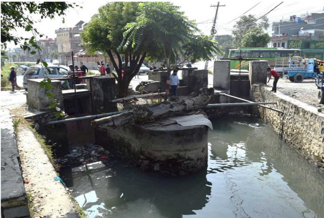
Figure 2: Bifurcation of canal into Irrigation Canal and Power Canal
