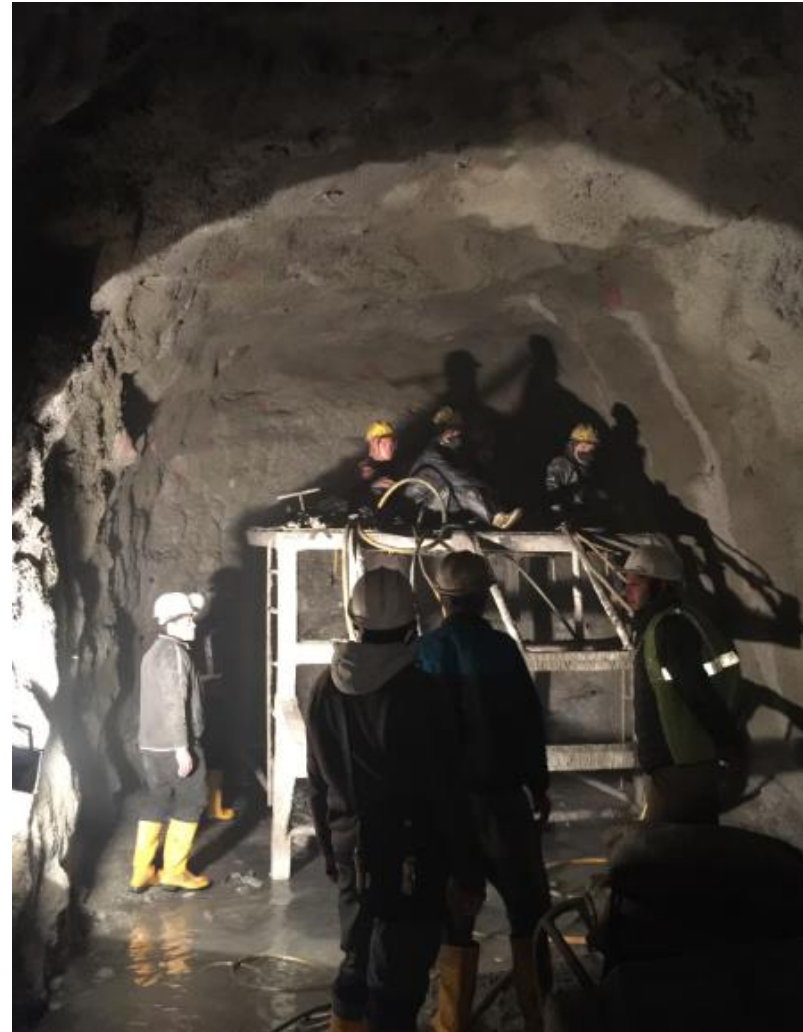
Shotcreting and finishing the excavated face
