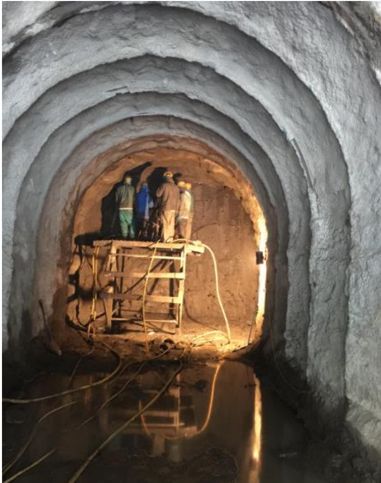
Support Installed in Headrace Tunnel
