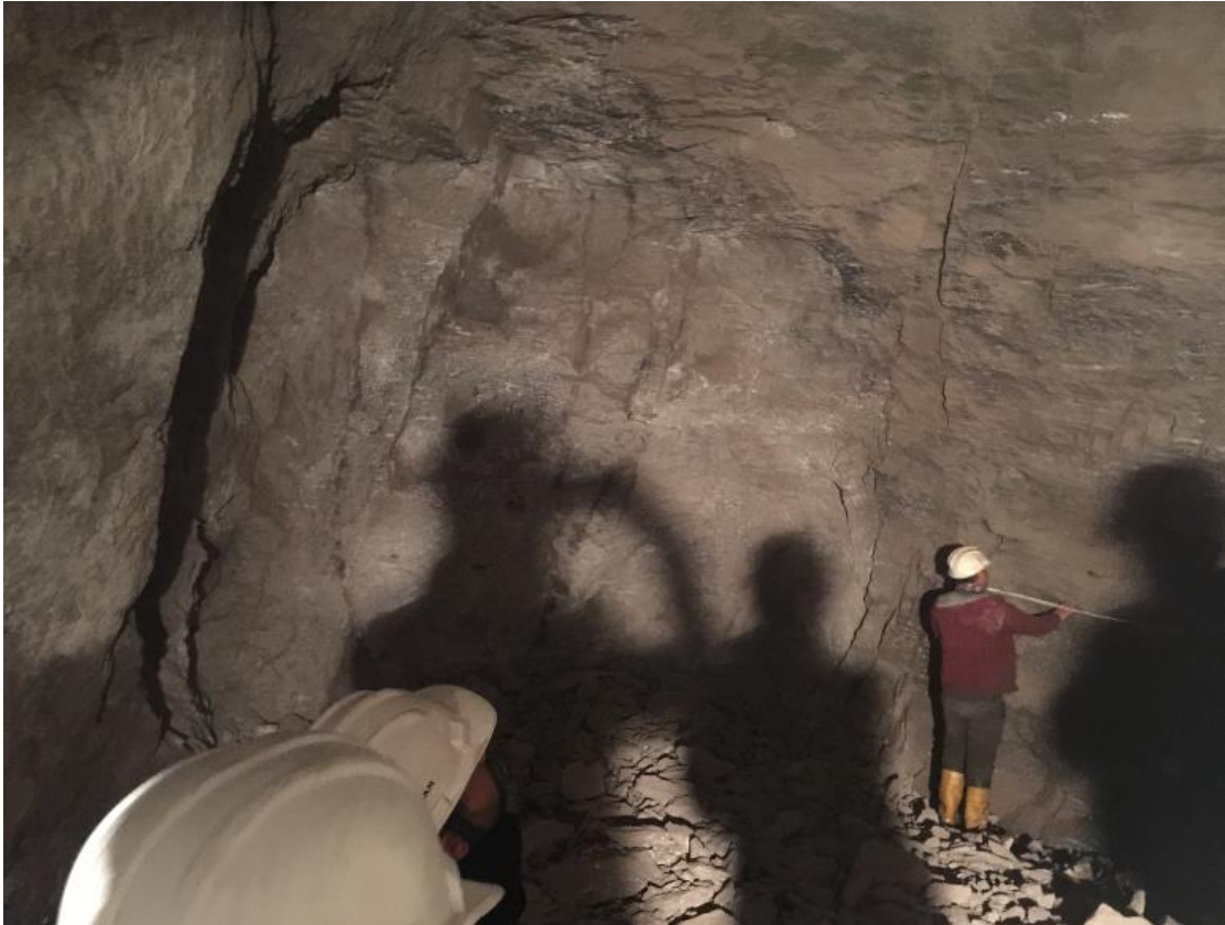
Measuring Joint Properties at the Tunnel Face
