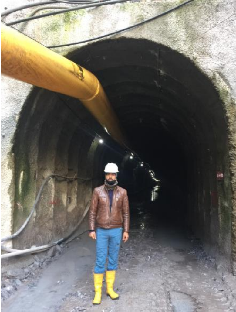
Portal of The Headrace Tunnel
