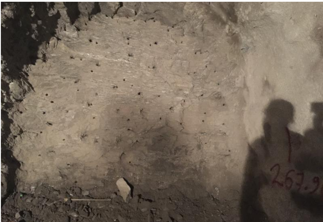
Drilling Pattern in face of Tunnel
