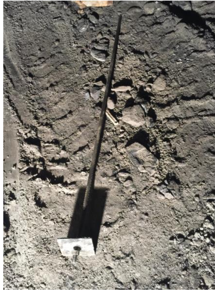
Sample of Rock Bolt used in the Site
