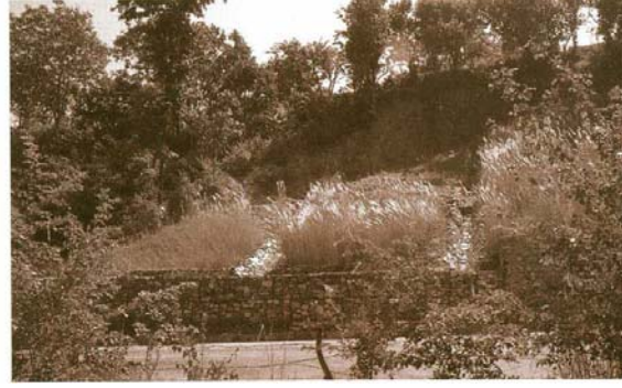
The same site, two years later, following establishment of the protective grass cover between the drains
