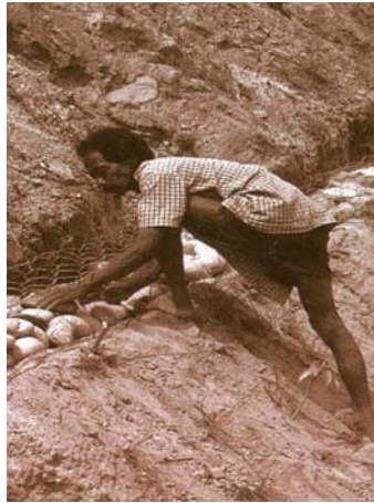
Figure 17: Construction of a wire bolster cylinder
