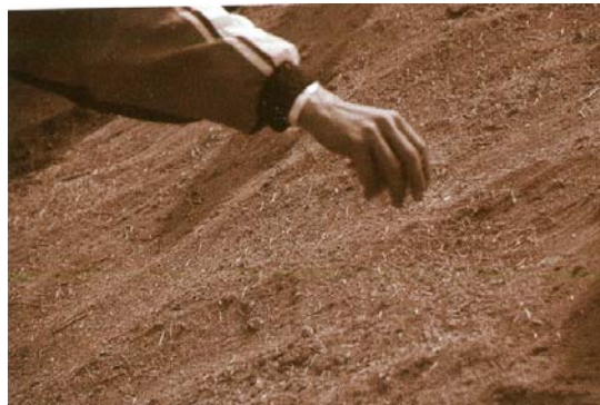
Figure 2: Grass seeding, the seeds or grass seed heads are spread liberally over the slope. Ideally, the whole surface should be very lightly covered in seed material.
