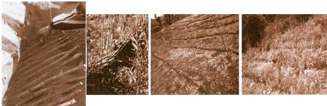
Figure 6: Brush layering- The first layer of cuttings is laid along the terrace, with a 50 mm interval between the cuttings( far left); a second layer of cuttings is placed on top (above left); layers are positioned at 1 to 2-metre intervals up the slope (above middle) and small terraces are developed in the long term (above right).
