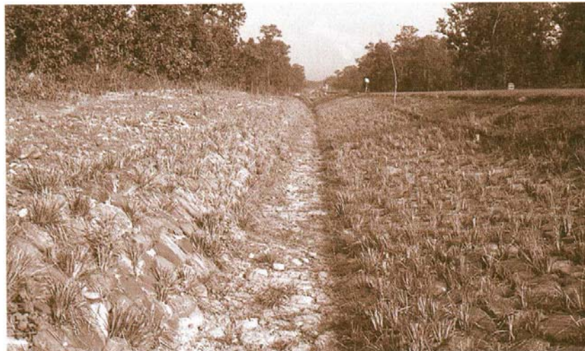
Figure 10: Vegetated stone pitching providing strong armouring
