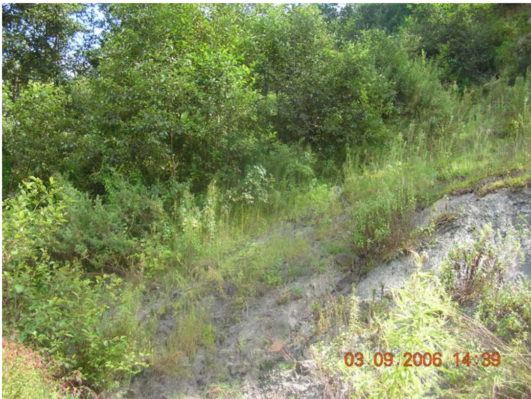
Figure 36: Tathali Phaidhoka Site showing the earth flow and vegetation
