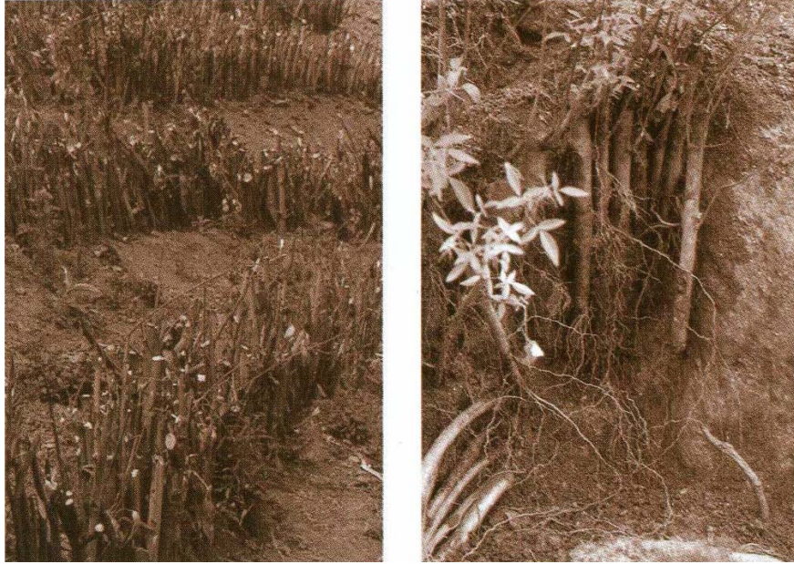
Figure 7: A completed palisade (left) and a Simali palisade excavated after one growing season to show the development of roots (right).
