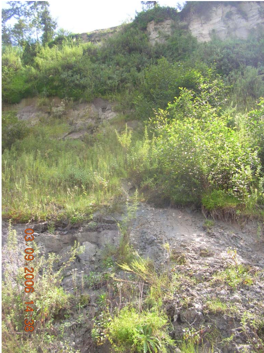
Figure 34: Tathali Phaidhoka Site showing the landslide and earth flow
