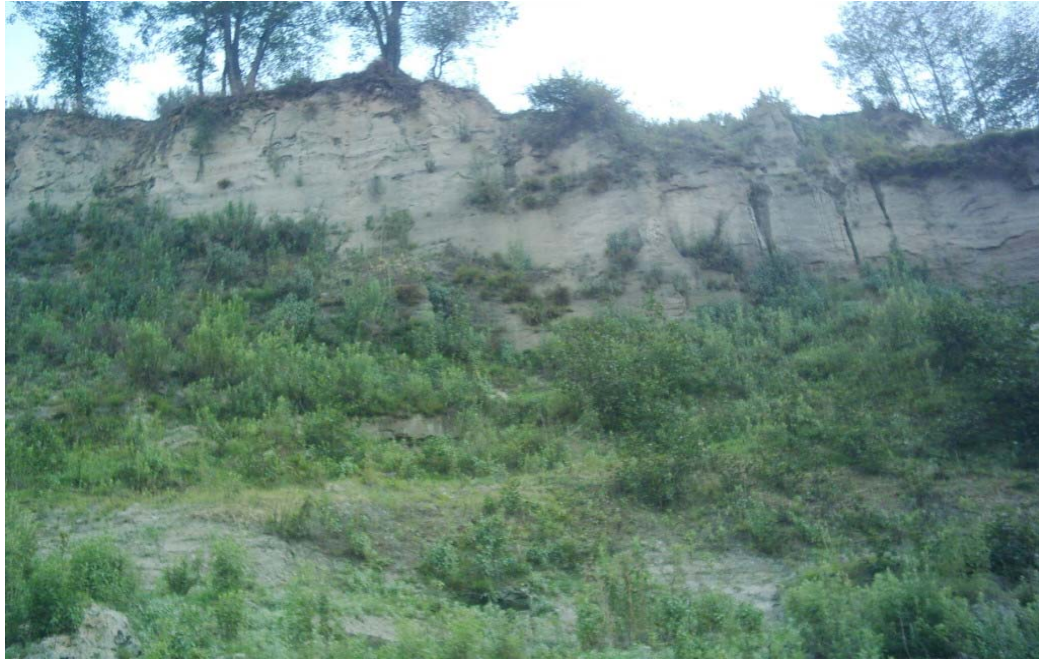
Figure 35: Tathali Phaidhoka Site showing the landslide
