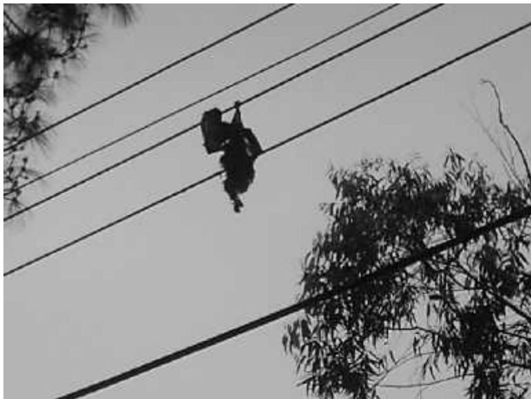
Photo 2: Dead bats hanging over electric wire
