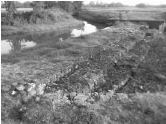
Picture showing the dam at Kesali river.
