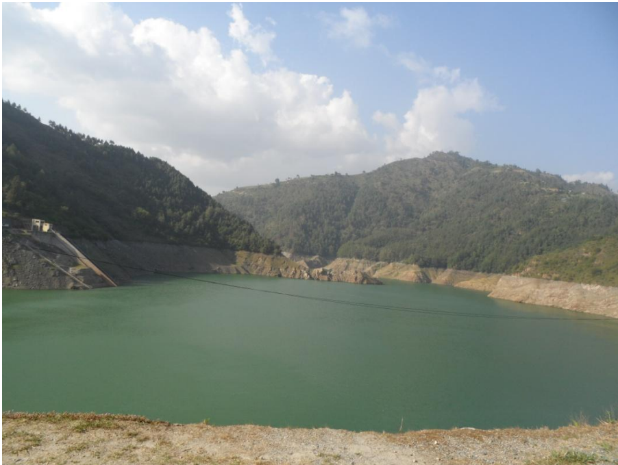
Figure 1.2 Kulekhani Reservoir with Sloping Intake (Source: (Manisamg, 2012))
