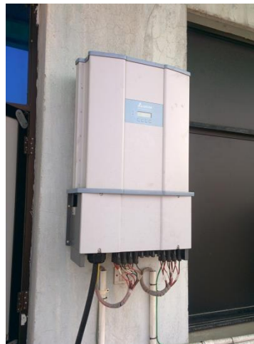
Figure 3-10: Inverter Installation
