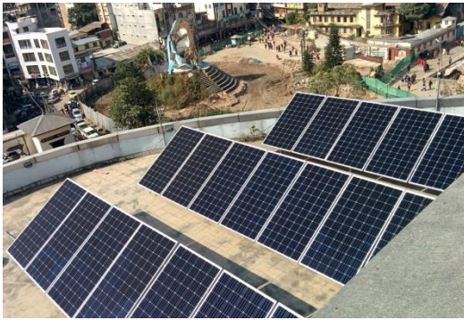
Figure 3-8: Roof 3-Solar Panel Installation
