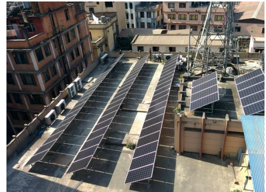
Figure 3-9: Roof 4-Solar Panel Installation
