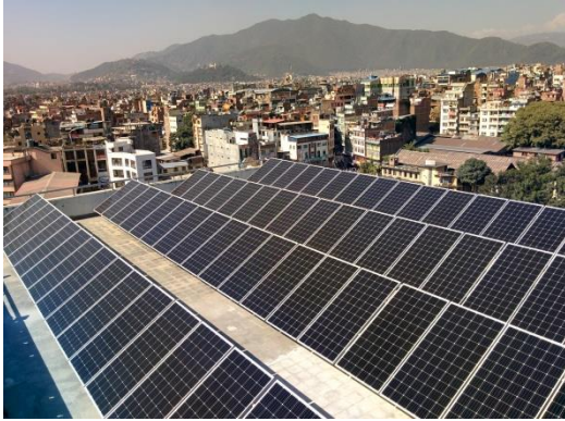
Figure 3-6: Roof 1-Solar Panel Installation
