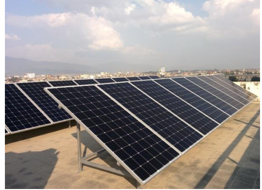
Figure 3-7: Roof 2-Solar Panel Installation
