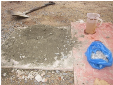
Concrete Mixing Process
