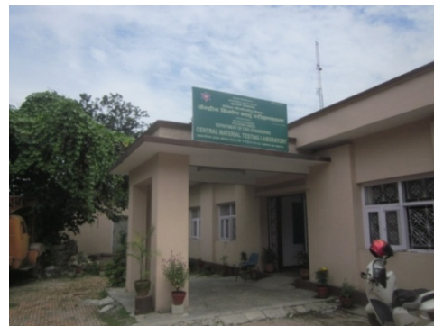
Central Material Testing Laboratory
