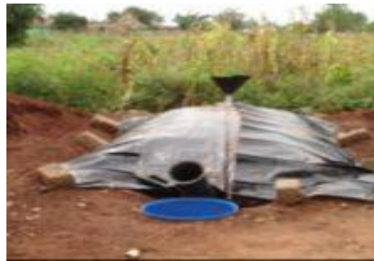
Fig: Ecofys Plastic Bag Digester.
