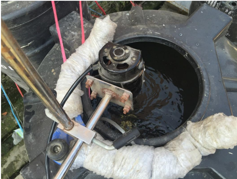
P6: Application of rotating pump in mixing
