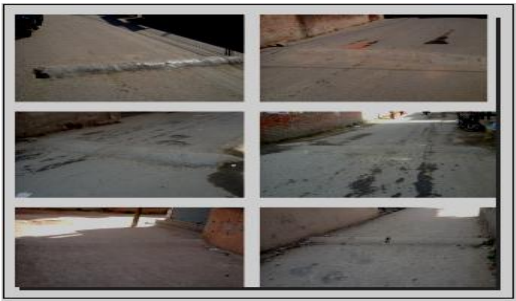
Figure 2.3 Un-uniformity in Hump Geometry Standard in Kathmandu Valley
