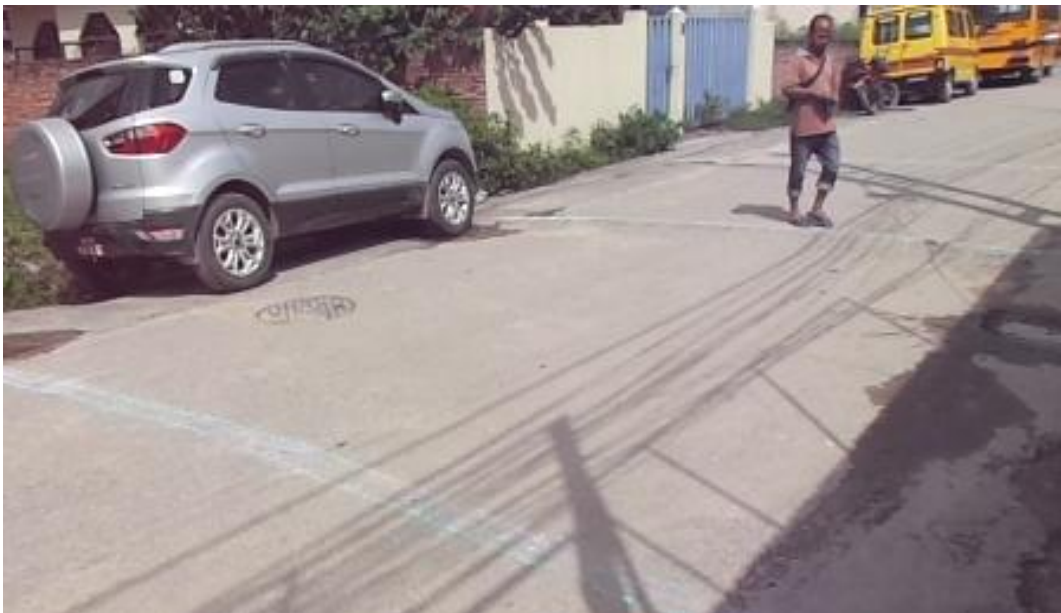
Figure 2 Picture at hump section of Buddhanagar site
