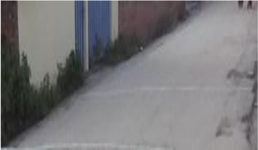
Figure 15 Picture at normal section of Buddhanagar
