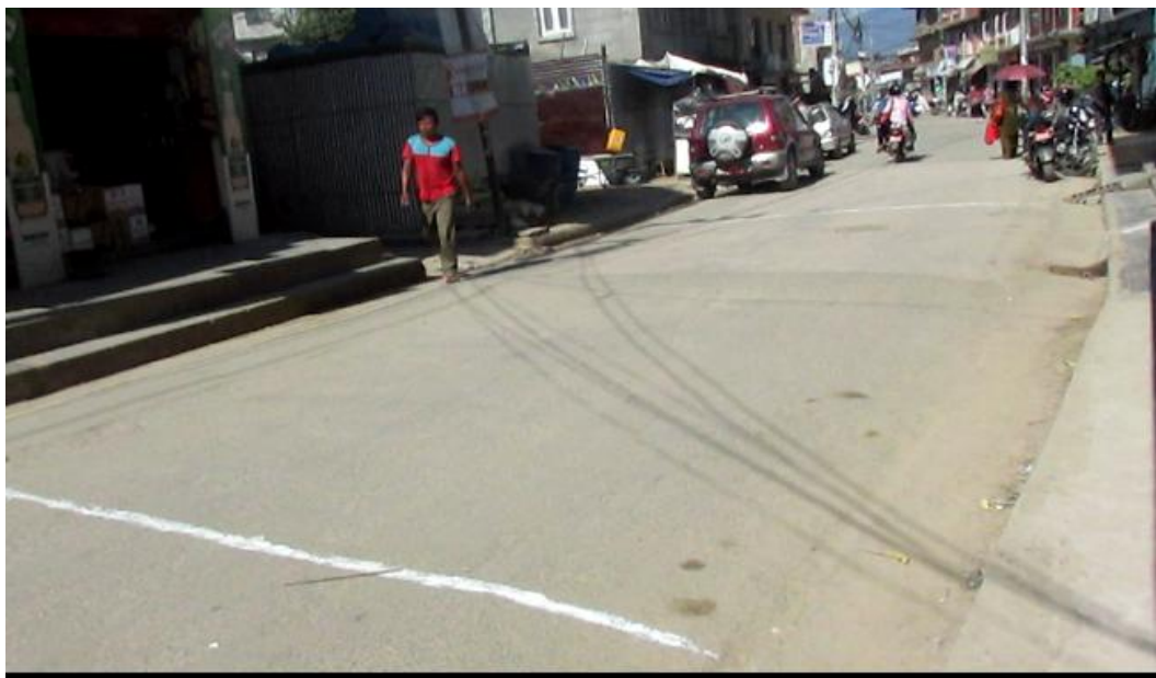
Figure 4 Picture at hump section of Talchikhel site
