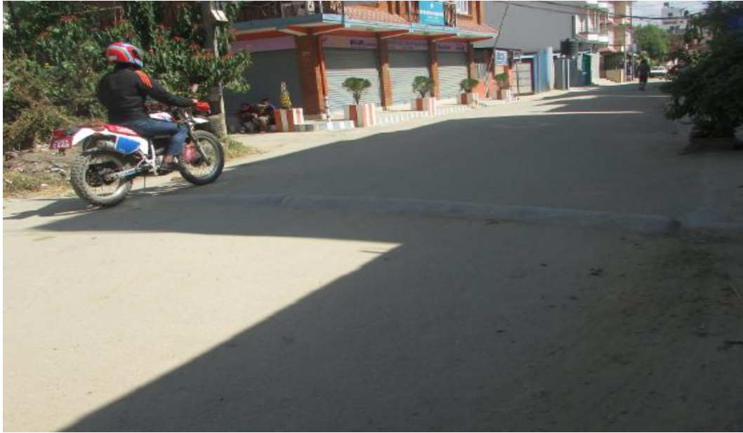
Figure 7 Picture at hump section of Bishalchowk site
