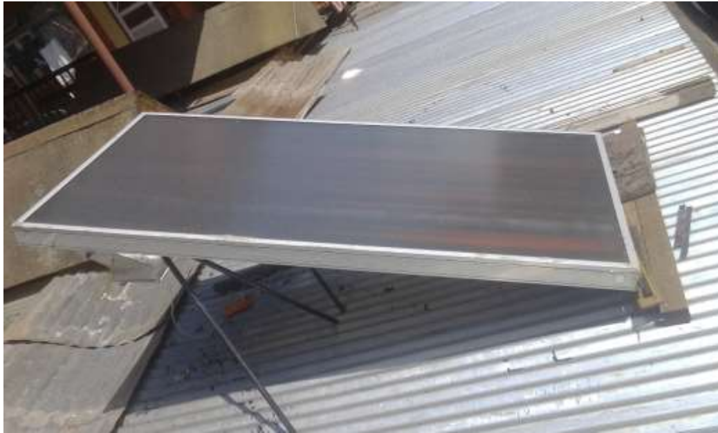
Figure 4.2 Staggered Type Solar Air Heater
