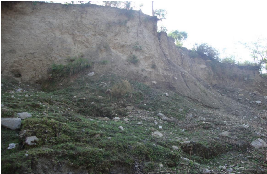
Figure 0.5 Close up view of Landslide area.
