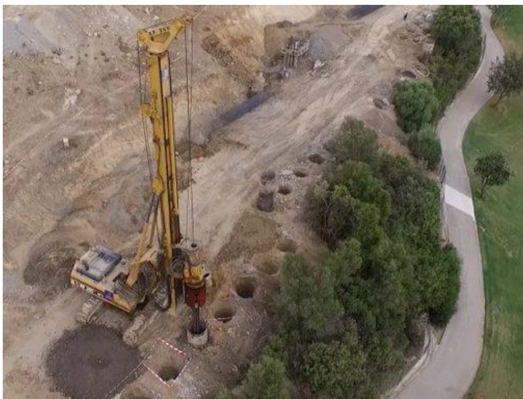
Figure 0.4 Slope being stabilized using concrete piles
