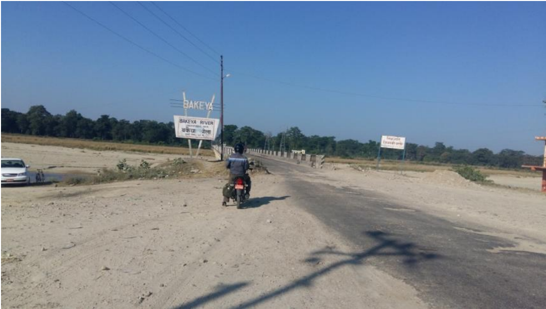
Photograph 3. A view near Lal Bakaiya Bridge.
