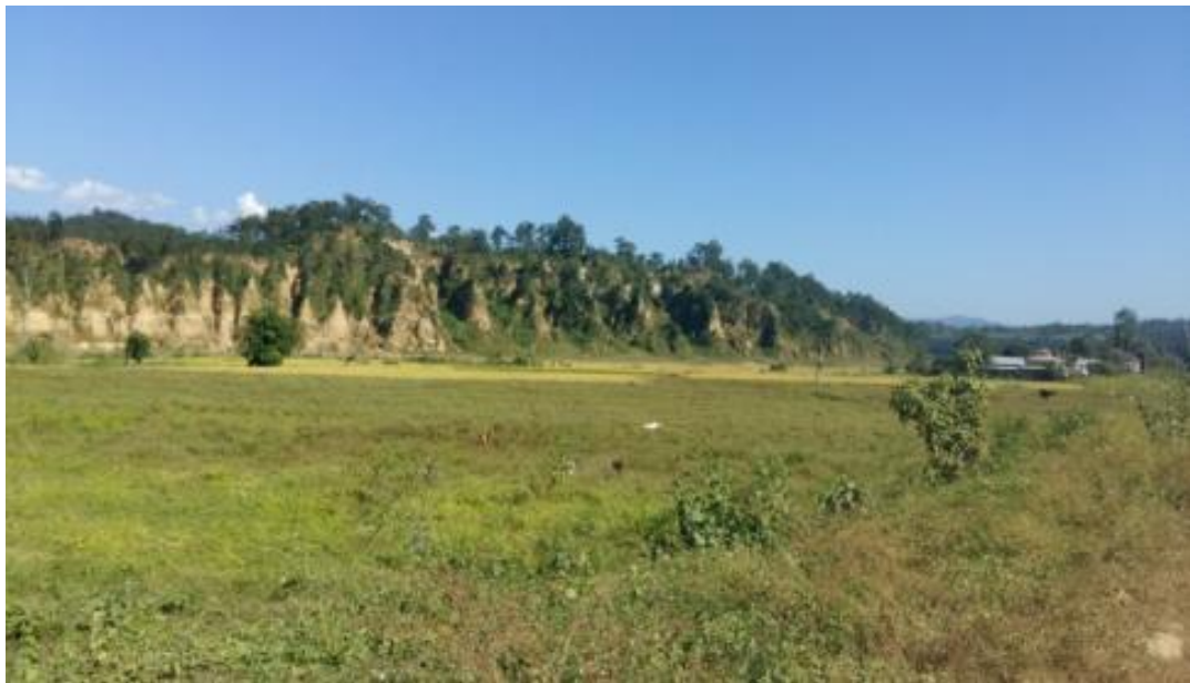
Photograph 8. Landslide observed near Shikharpur in the watershed.
