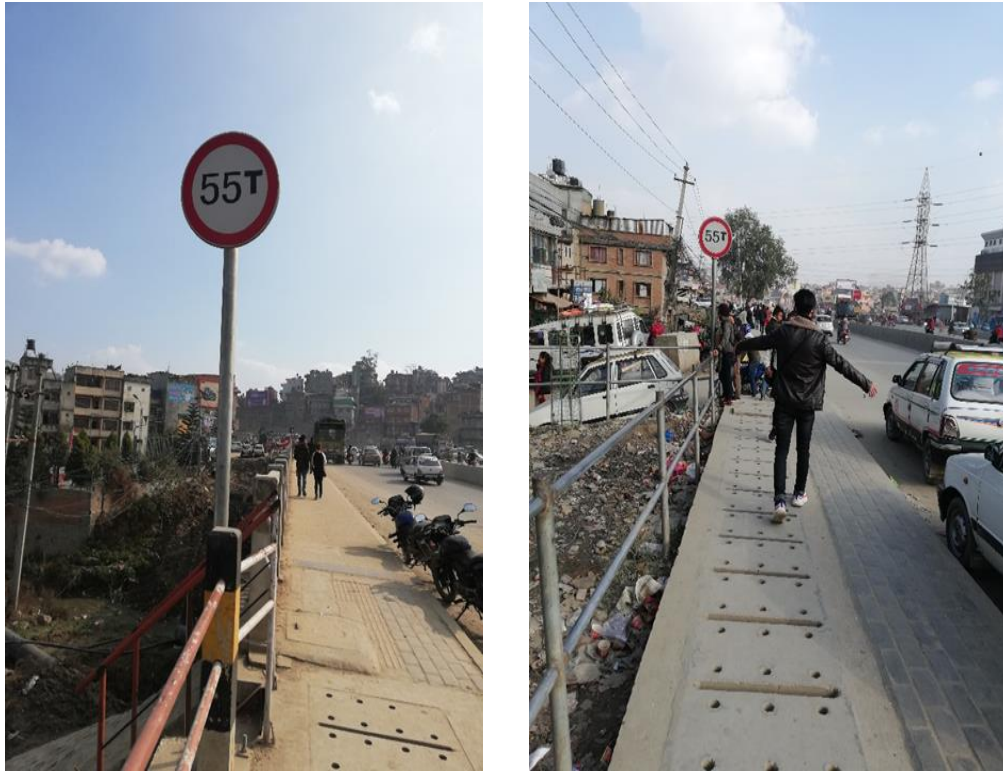
Figure 4.7 Khasibazar and Balkhu Bridge
