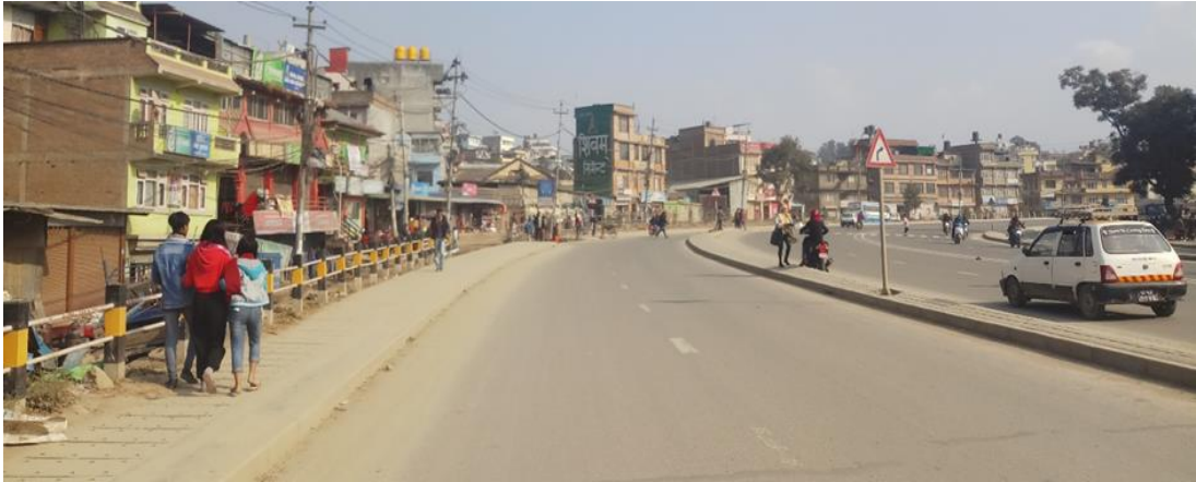
Figure 4.5 Horizontal Curve at Sanepa
