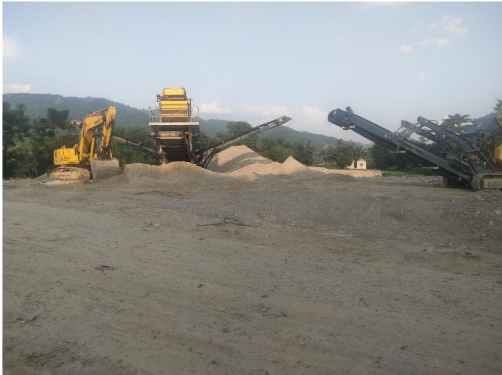
Figure 1.3: Crusher plant of Bagmati River
