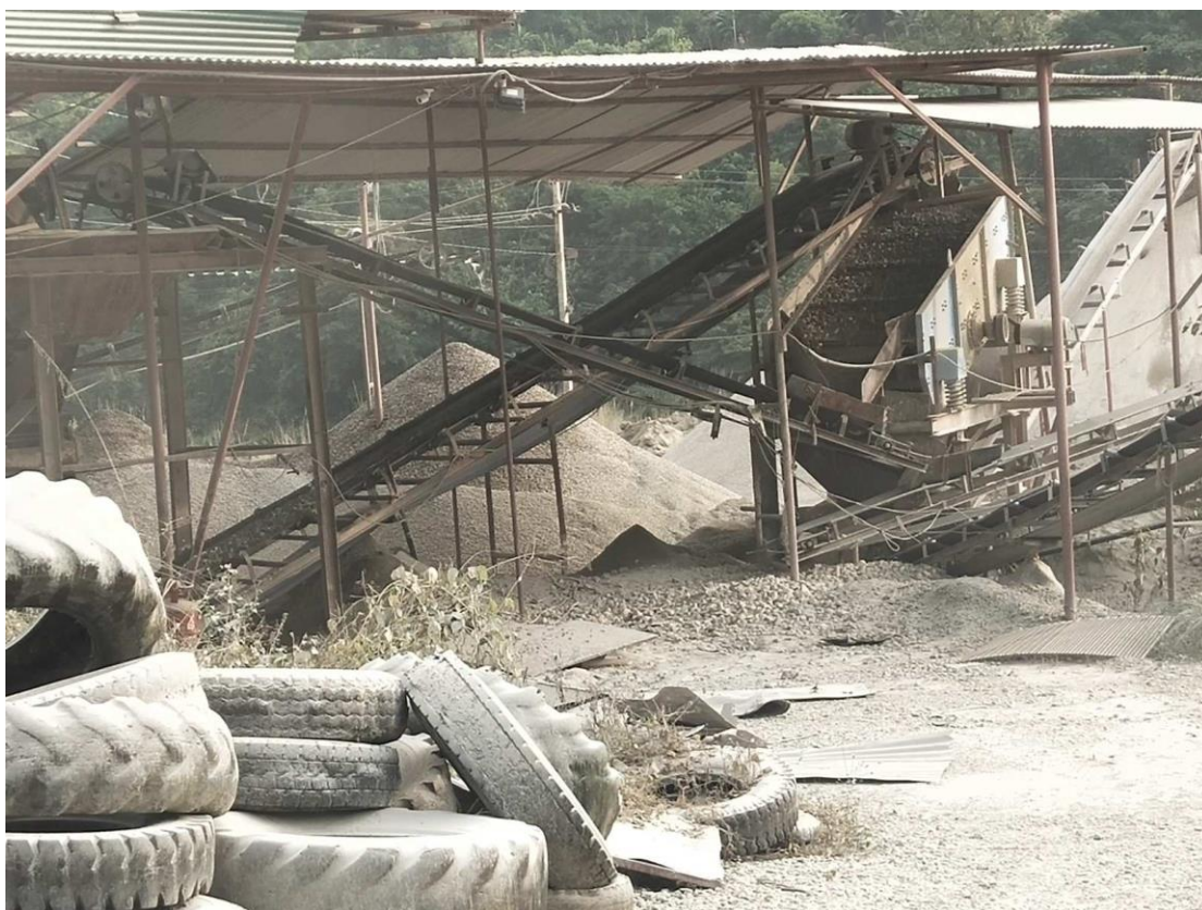
Figure 1.5: Crusher producing crushed aggregate from natural aggregate
