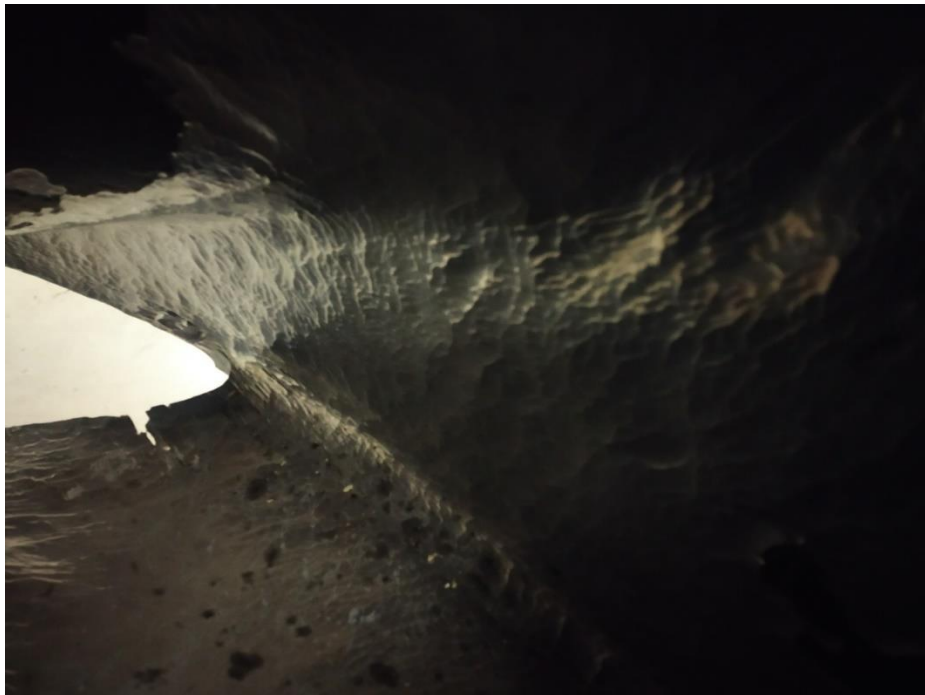
Figure A.6: Tear detected in the outlet side of runner blade
