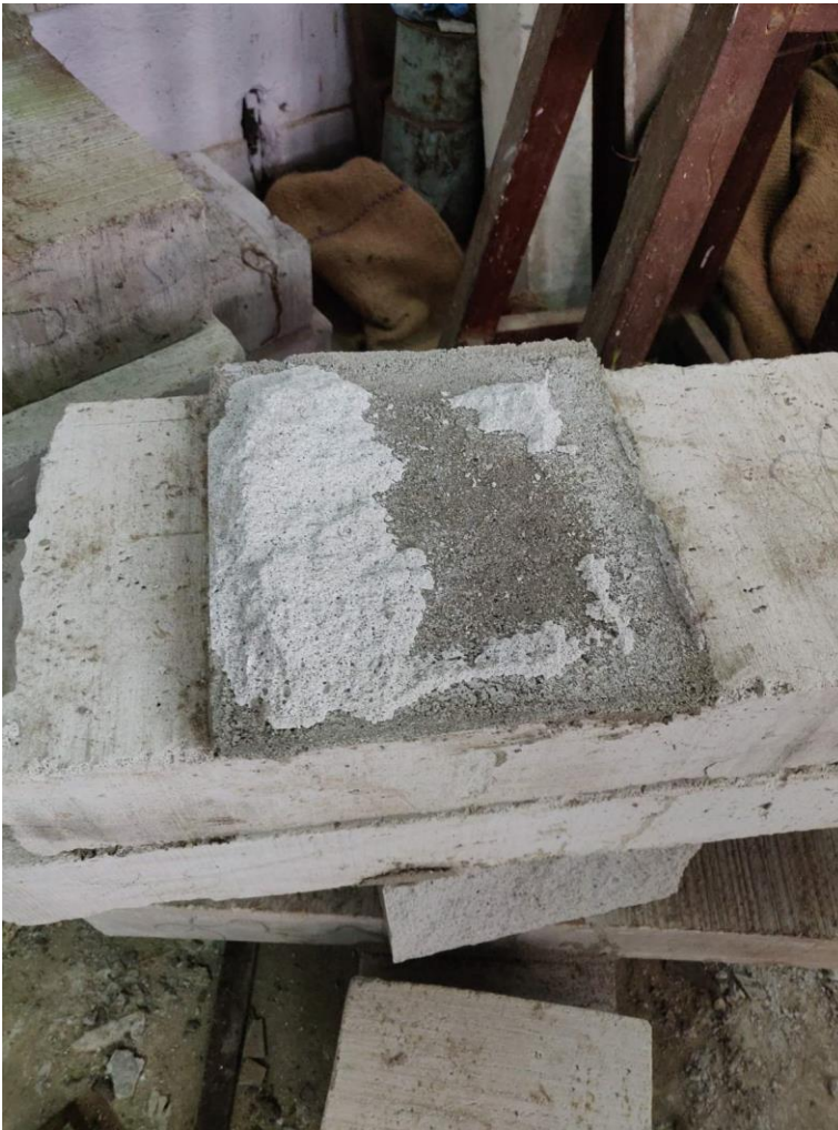
Figure 26 Partial block-mortar interface failure (Type II)
