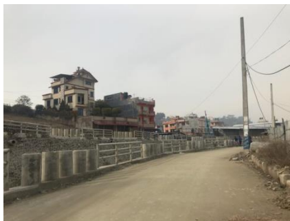
Image 4 Dhobikhola corridor: Flood plain and liquefaction area
