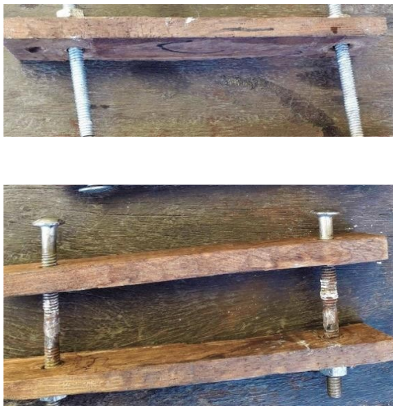
Figure 3.4: Fixing nuts and bolts
