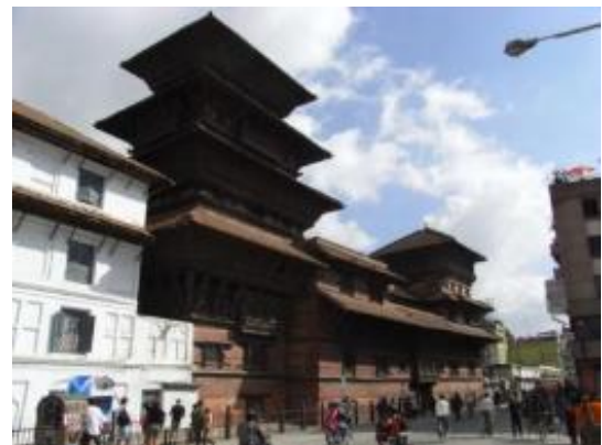
Figure 12 Landmark L2 - Nine Storey Palace Tower
