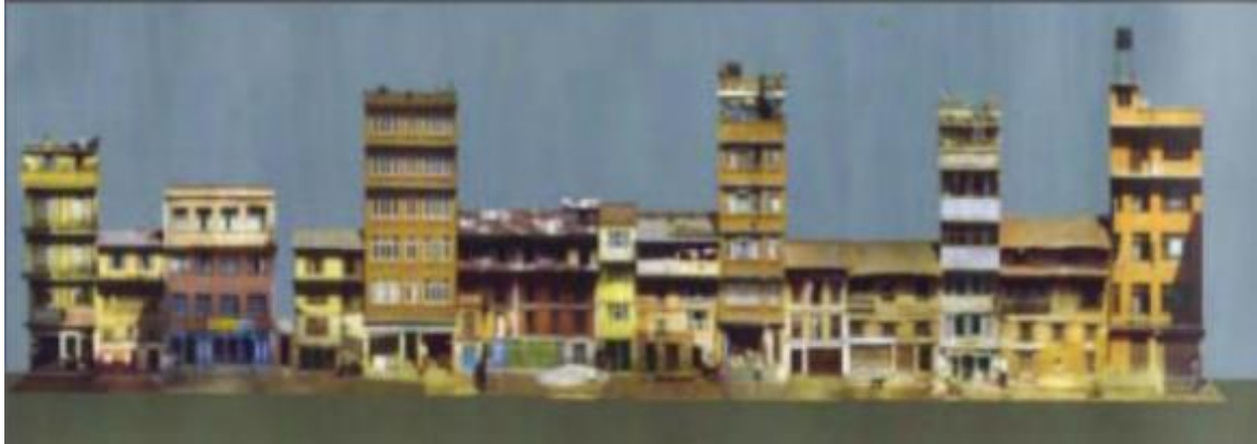
Figure 30 Impact of planning bylaw on street elevation (source: The P.U.S.H Effect, People, Urban, Society and Heritage , Rakshya Rayamajhi)
