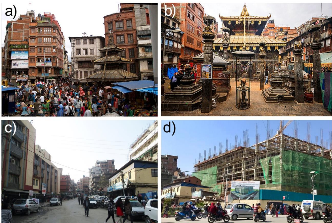
Figure 7 a) Ason b) Jana Baha at Keltole c) Towards Mahabouddha from Kanti path d) Under construction surgical block of Bir hospital.
