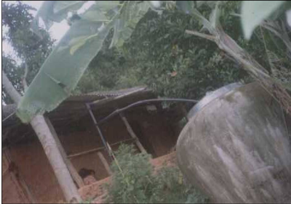
Photo 3: Corrugated Galvanized Iron water harvesting
