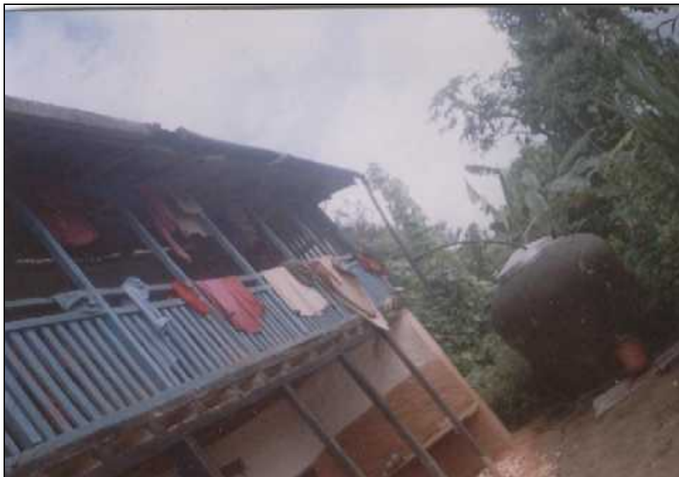
Photo 4: Roof top CGI water harvesting system
