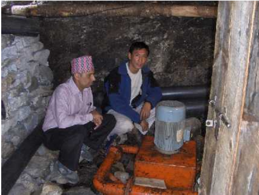
The researcher observing a peltric set installed in a stream located near Monjo.
