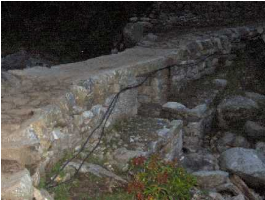
The people leaving near Monjo have constructed a bridge by using only stones.
