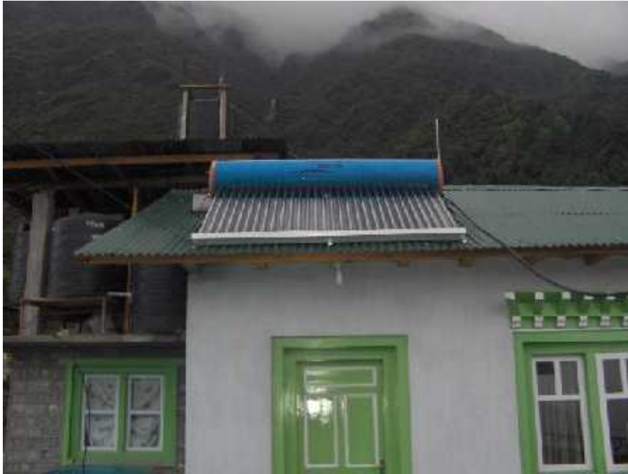
A tourist standard hotel at Lukla using solar power for both lighting and water heating.
