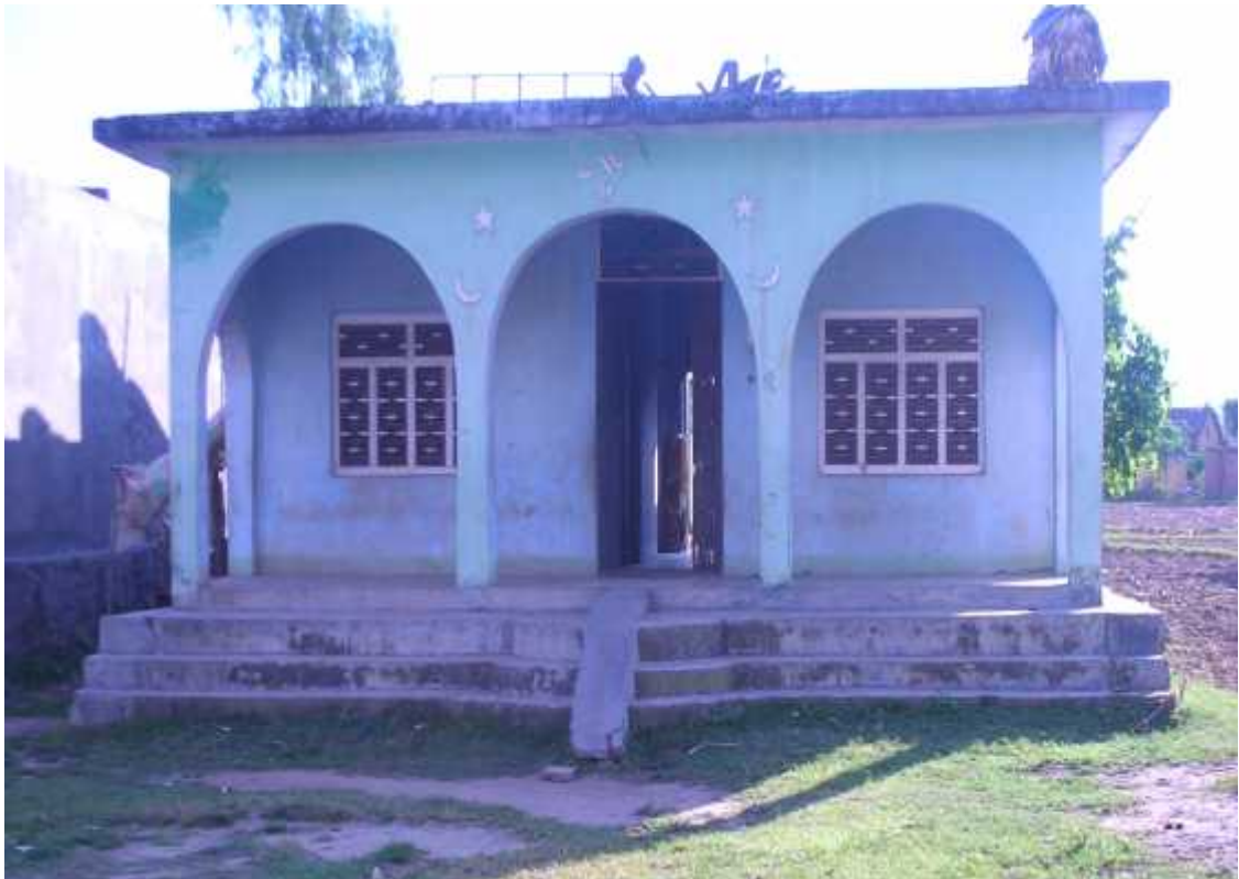
A RCC House of a Respondent in the Study Area.
