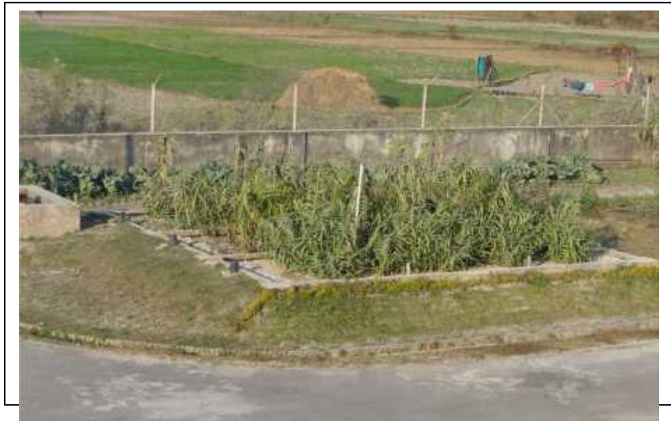
Photo 1: Overall view of Horizontal Flow Constructed Wetland.
