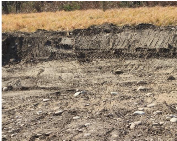
Photo 11 Artificial waterhole construction inside the Park
