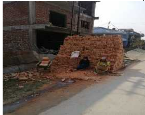
Figure 5 Women doing labour job for house construction
