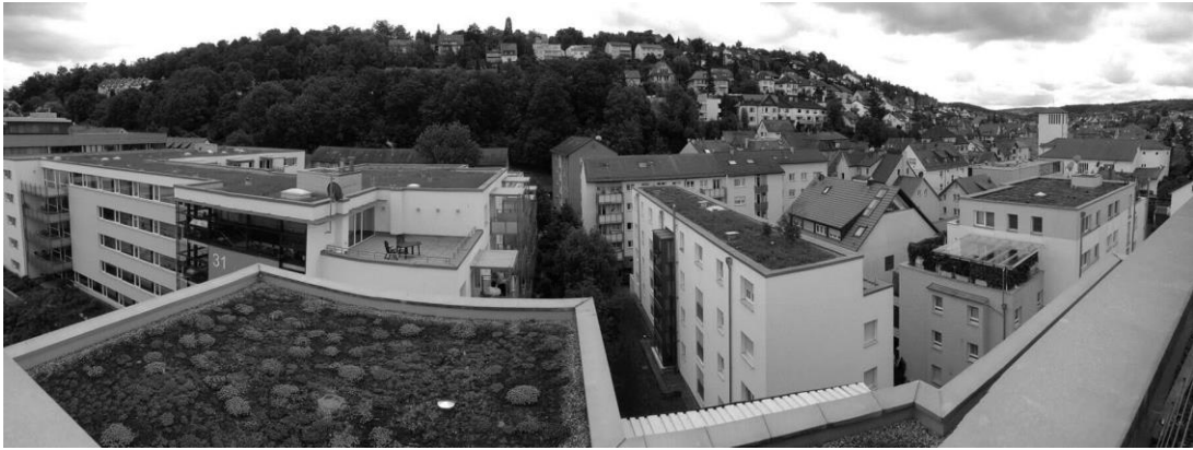
Figure 18 Green roofs in Stuttgart
