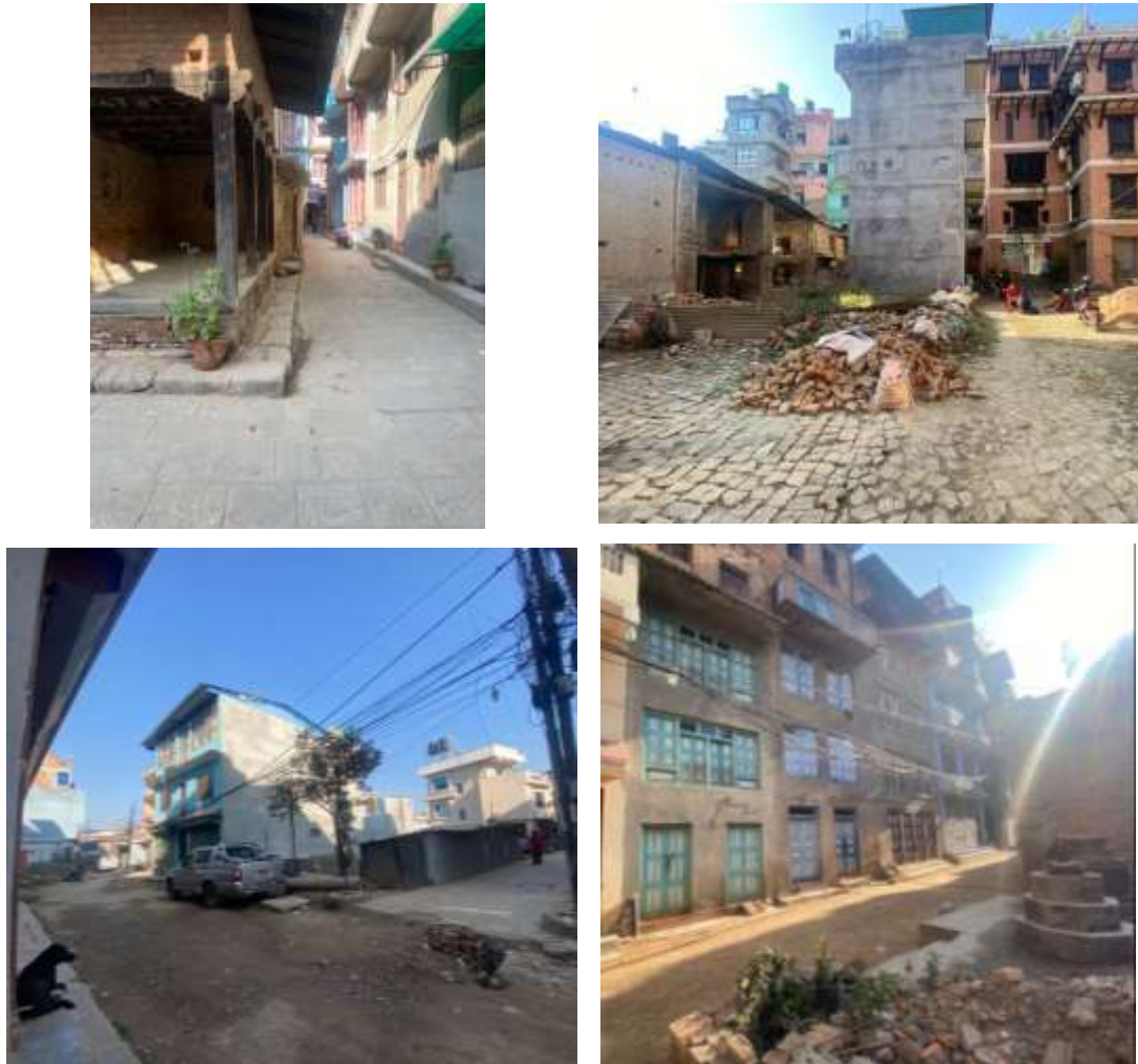
Figure 43: Various Pavements across different locations
