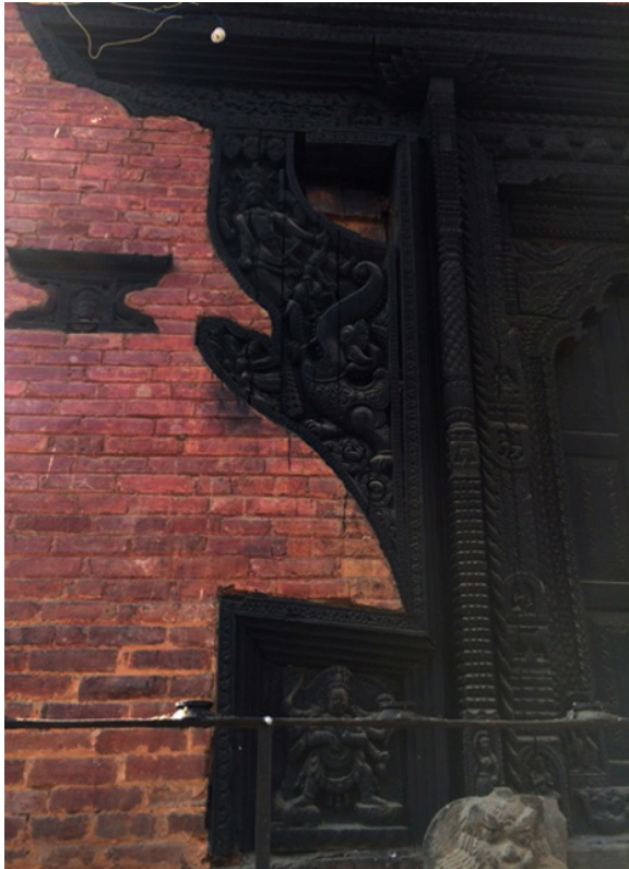
Figure 46: East door of the main shrine
