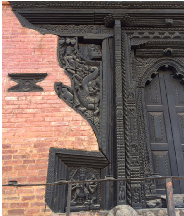
Figure 44: North door of the main shrine
