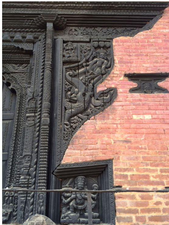
Figure 47: East door of the main shrine
