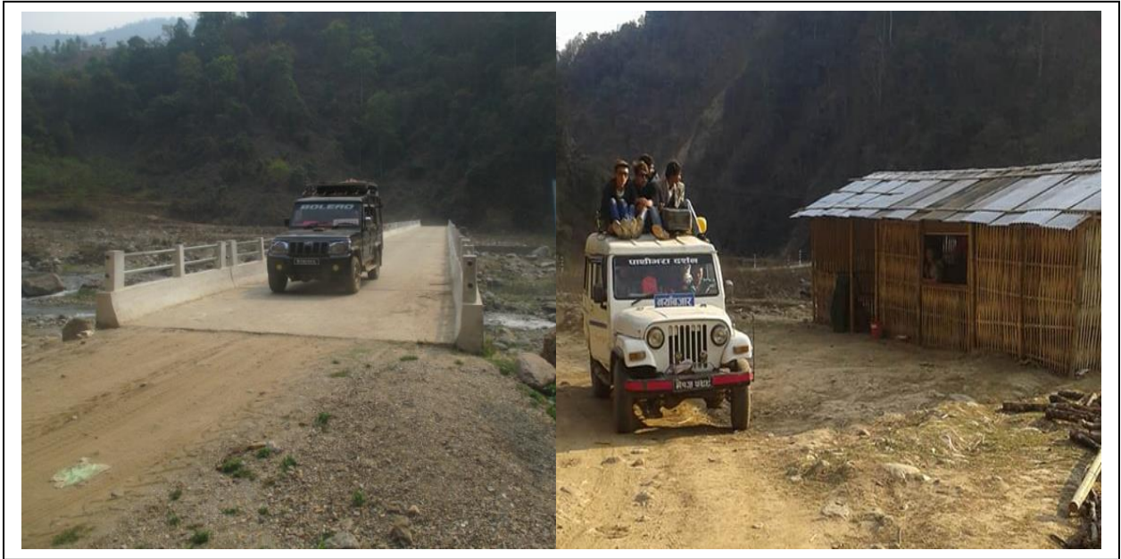
Public vehicles are plying over the Mai Bridge and its roads alignments.
