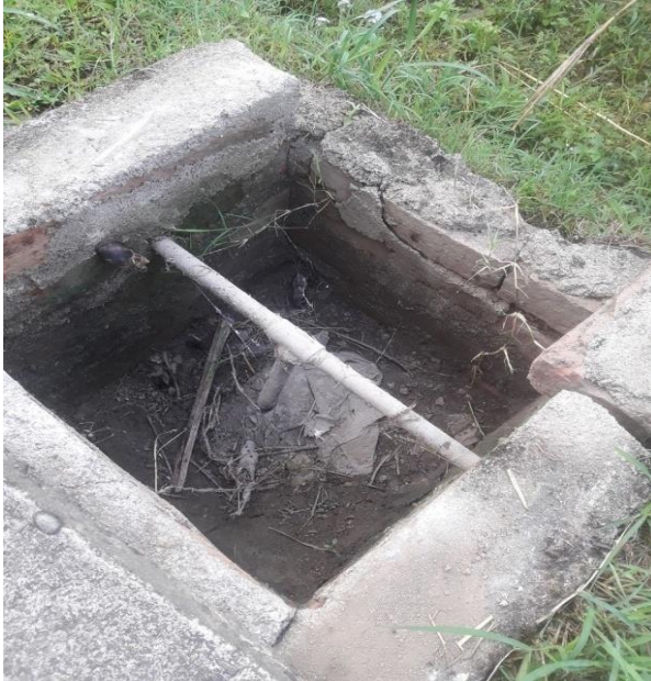
Picture - 2: 8 m 3 Biogas Plant
