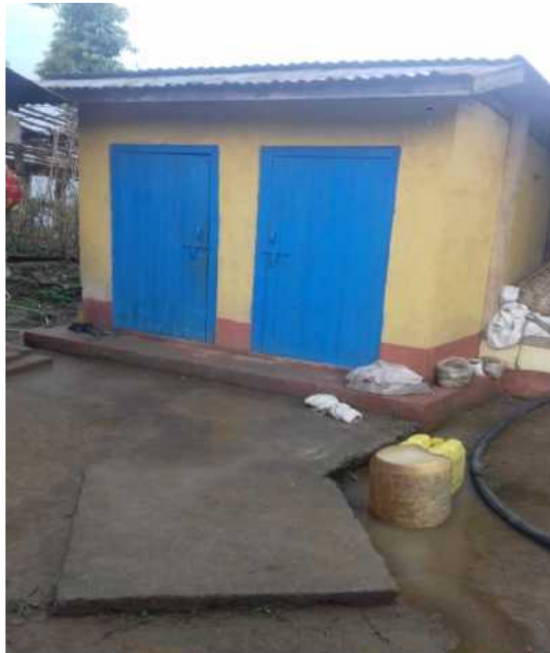
Cemented House and Toilet of Respondent Family
