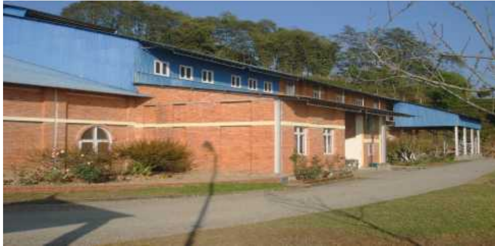
Picture: Factory building view
