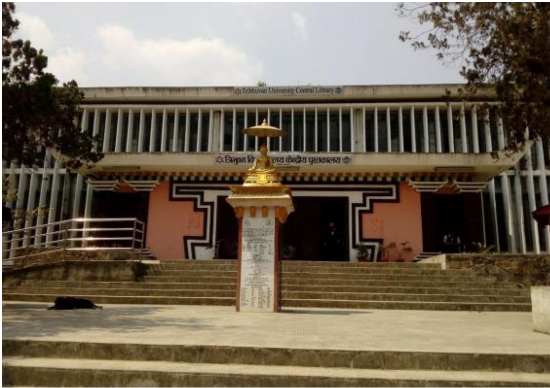
Figure 46: Front View of Library
