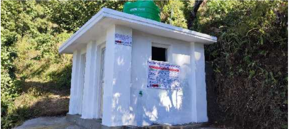
Photograph of School Toilet Constructed by the Program
