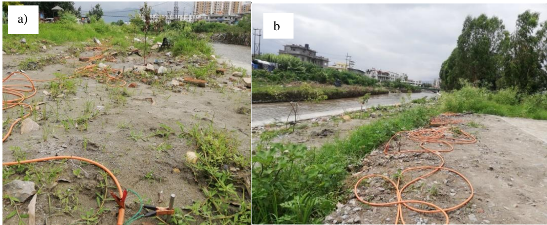
Figure 73: Photographs of MW10 profile a) towards first electrode, upstream and b) towards last electrode, downstream
