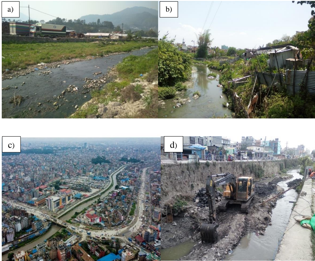
Figure 13: Sediment pattern along the Bishnumati River a) Channel material at upstream section b) Channel material at downstream section c) Channelization, dense settlement and road along river, source-Setopati.com and d) River training works in river channel
