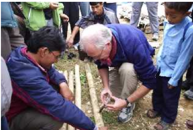
Treatment of bamboo by using chemicals
