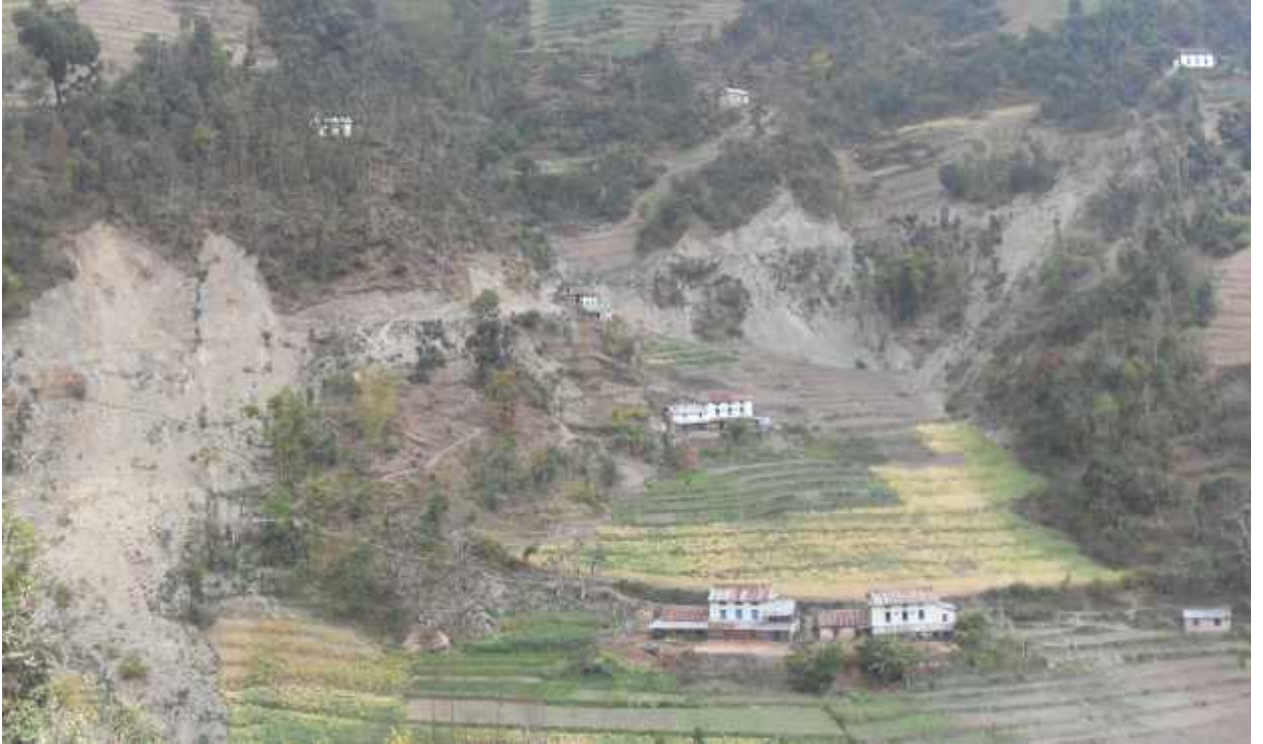
Photo 1: A photo showing the Peltric set house, pipe line lay up to Peltric set house, and nearby houses.
