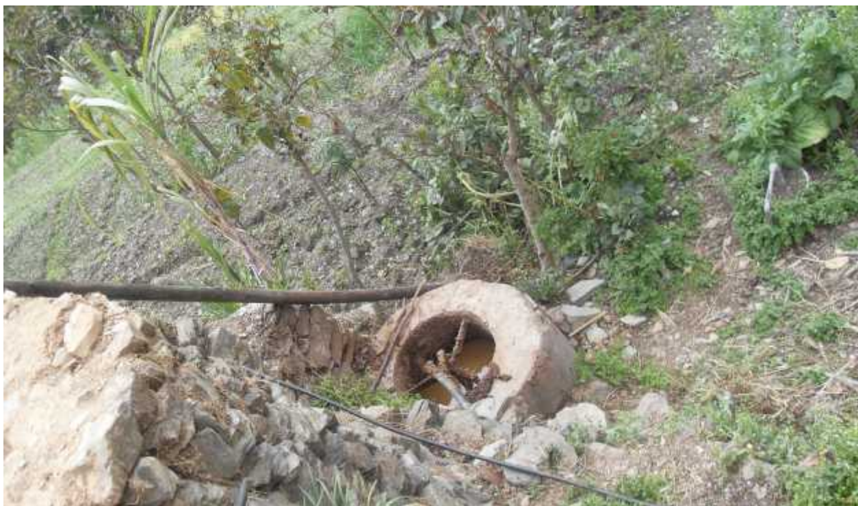
Photo 5: A Gobar gas plant at Ram Chandra Chaulagain's house. It is used for cooking purpose.
