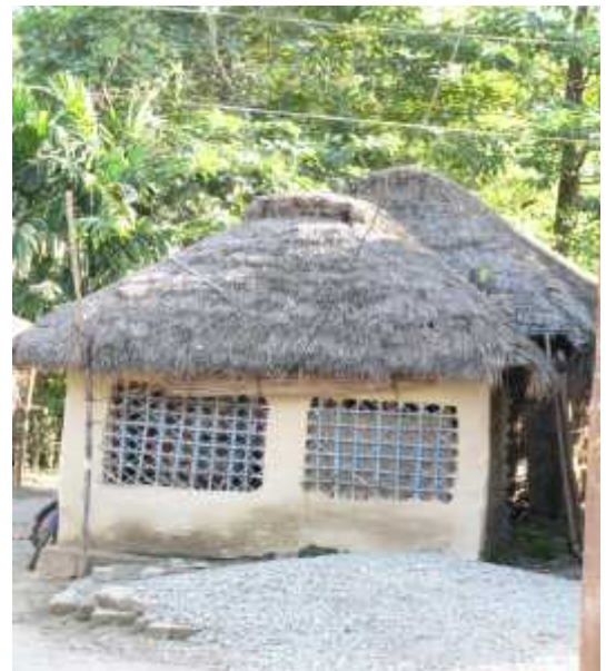
Photograph 10. Local type of building of Madhesi Indigenous (Inaruwa municipality)
