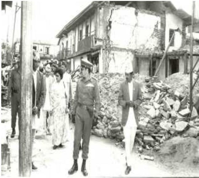
Photograph 4. 2045 Earthquake in Nepal
