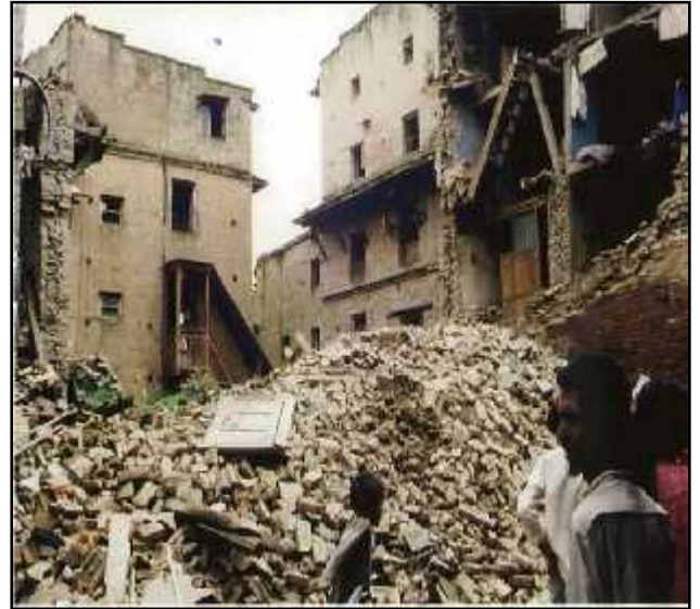
Photograph 5. 2045 Earthquake in Nepal
