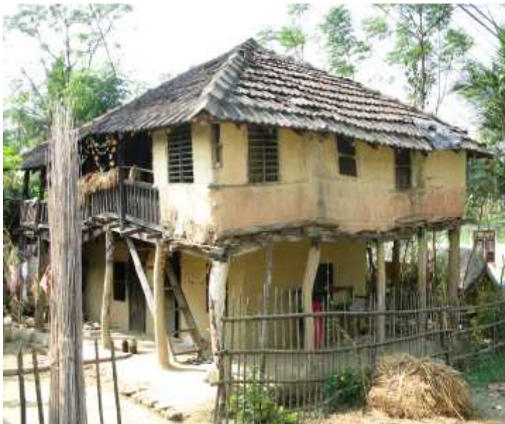
Photograph 9. Vulnerable Building (Inaruwa municipality)
