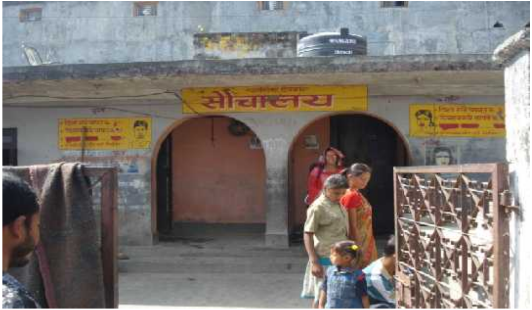
Some Photos about the Condition of Public Toilet.
