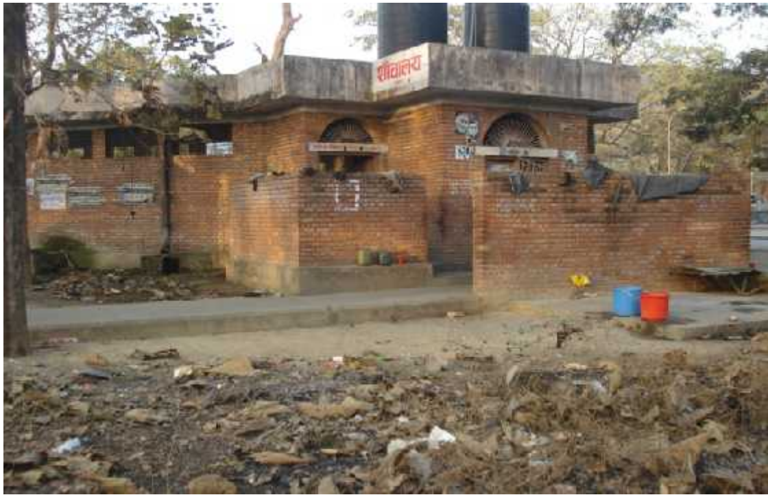
Photo No. 11: Surrounding Area in Bus Park Public Toilet.
