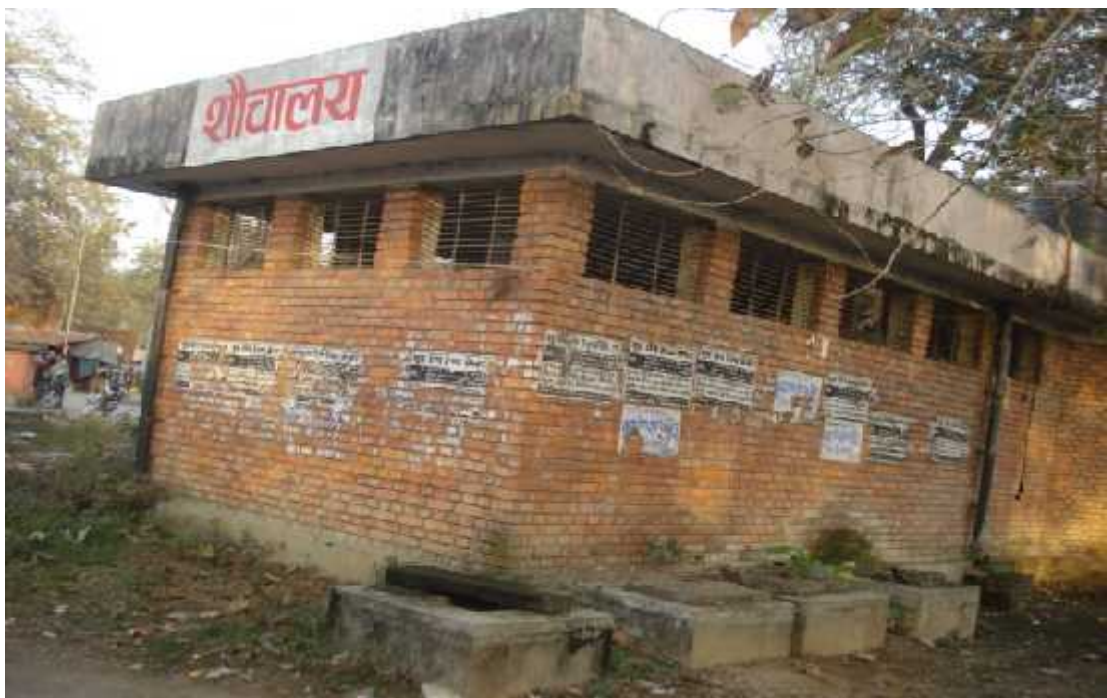
Photo No. 1: Public Toilet in Haat Bazar
