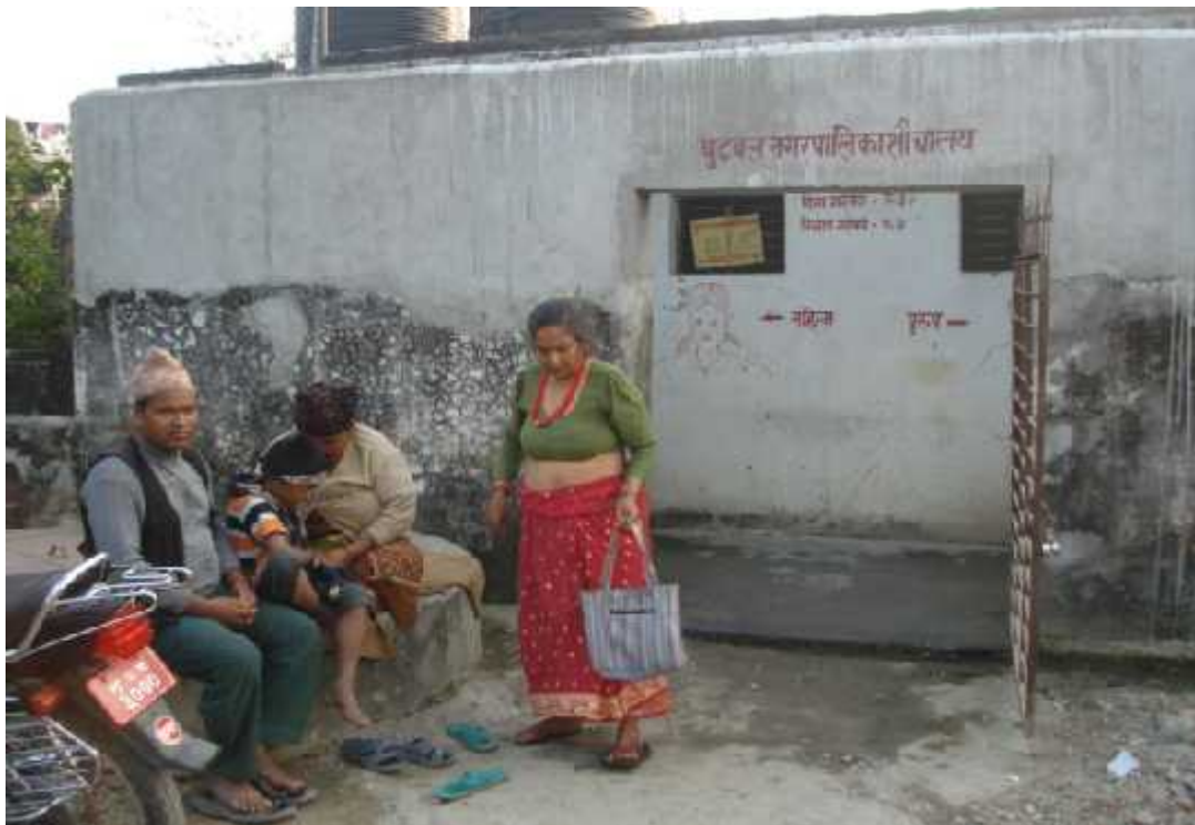
Photo No. 10: Fee Collector in Devi nagar Public Toilet.
