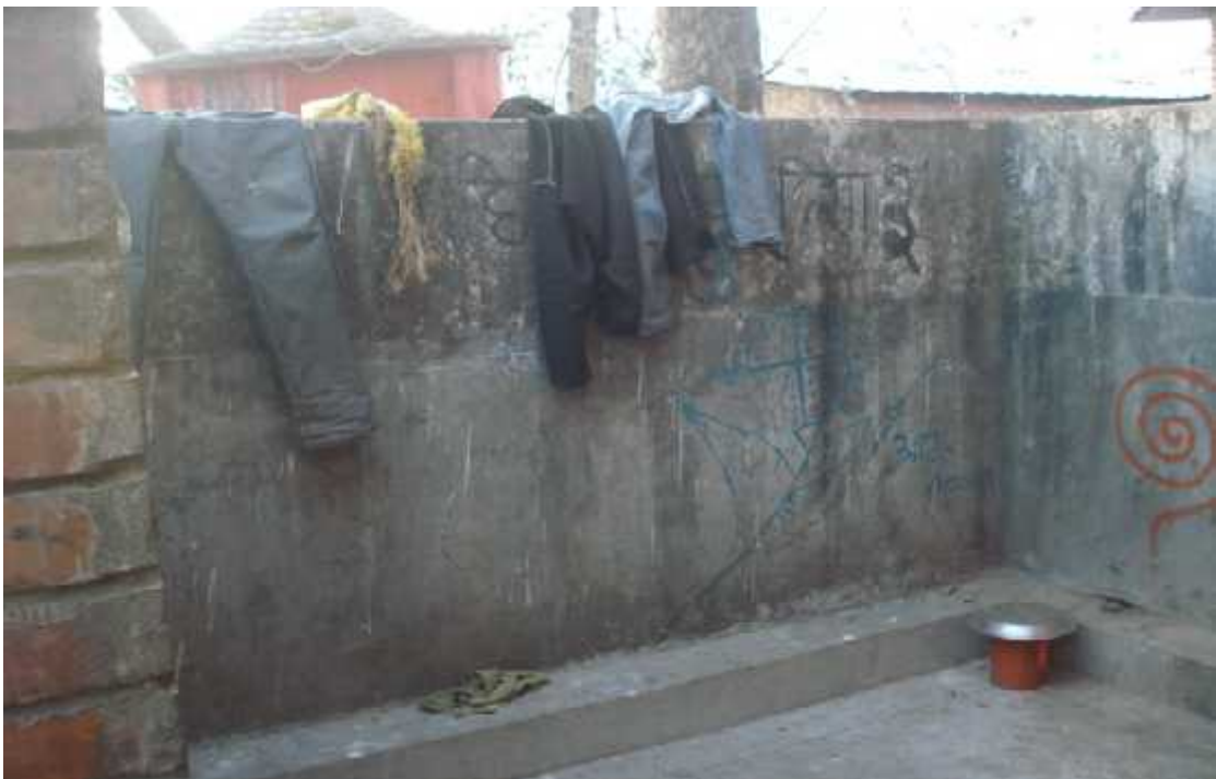
Photo No. 6: Surrounding Area of Haat Bazar Public Toilet.
