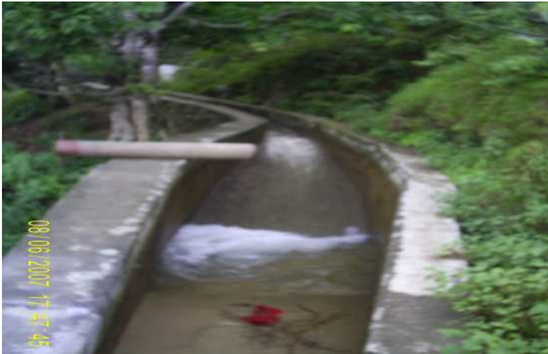
Cannel to supply water
