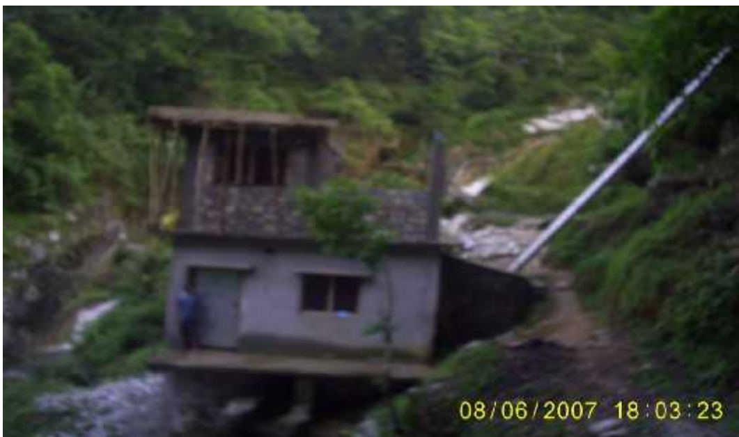
Power house of the Putputte Hydro-project
