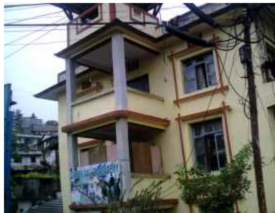
Photo 5.4: Electric Network in Ilam Bazar
