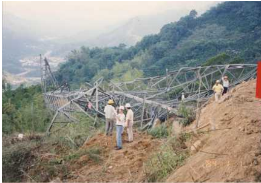
Photo 2.3.3: Electric Tower Damaged By Earthquake Shaking
