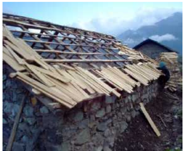
Plate 4: A house being roofed with the wooden tiles.
