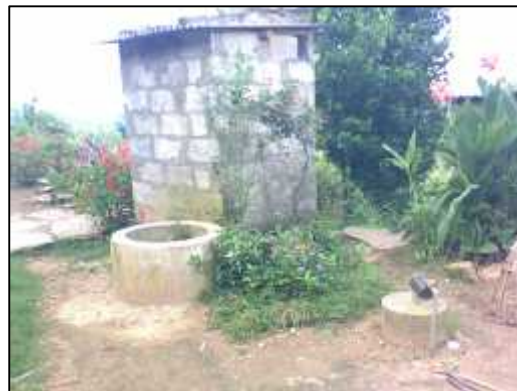
Toilet attached Biogas.
