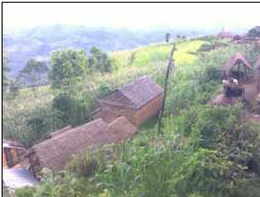
Distribution line of MHP in study area.
