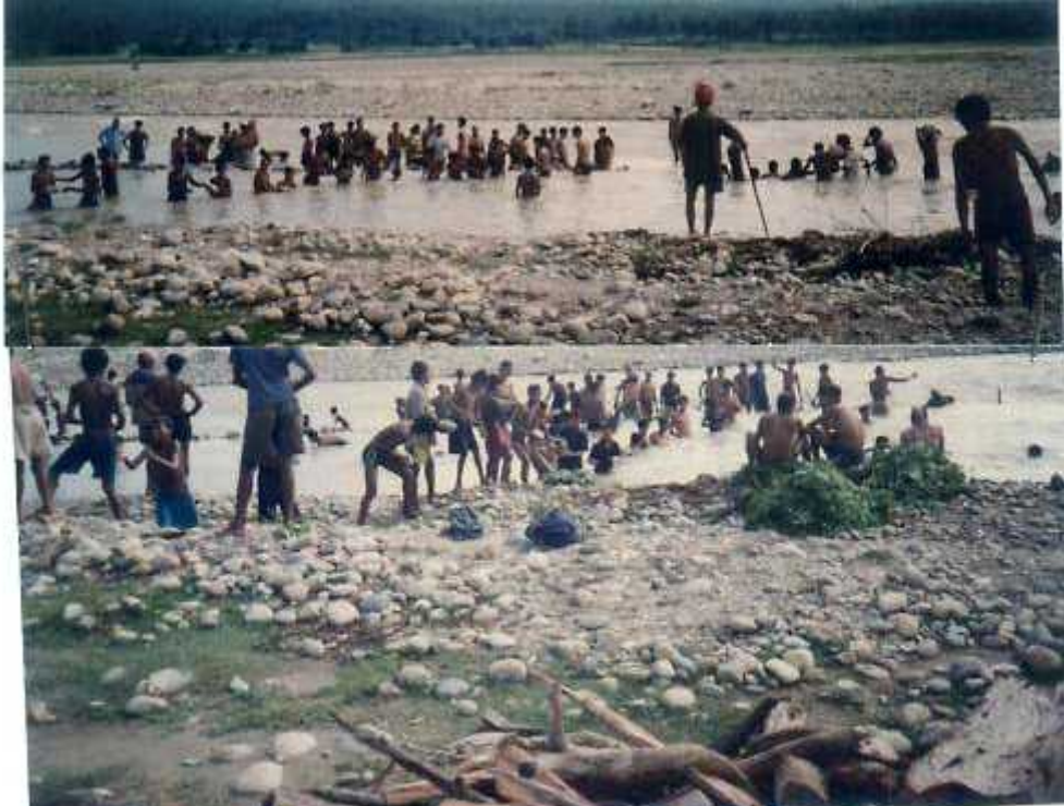
Photograph 3: Participation of villagers to make 'Kulo' (dam) on the Kamala river. Danuwar Metha is standing with stick and ordering everyone.
